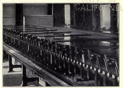
Courtesy of the "Railroad Age.Gazette" THE ELECTRO-PNEUMATIC SIGNAL-BOX IN THE CONTROL TOWER OF A MODERN TERMINAL
