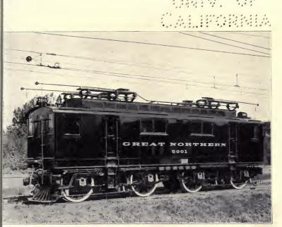
TRIPLE-PHASE ALTERNATING-CURRENT LOCOMOTIVE BUILT BY THE GENERAL ELECTRIC CO. FOR USE IN THE CASCADE TUNNEL, OF THE GREAT NORTHERN RAILWAY
